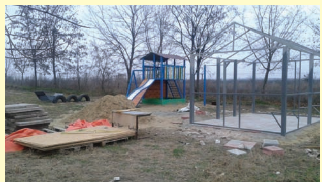
Work at the playground in progress
